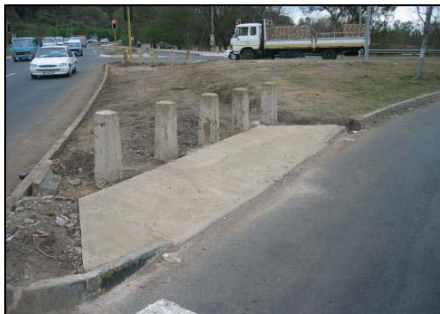
Closely spaced bollards at Camps Drift intersection during construction
