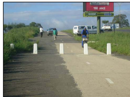
High speed section along old service road. Note bollards to prevent use by vehicles along the full length of path.
